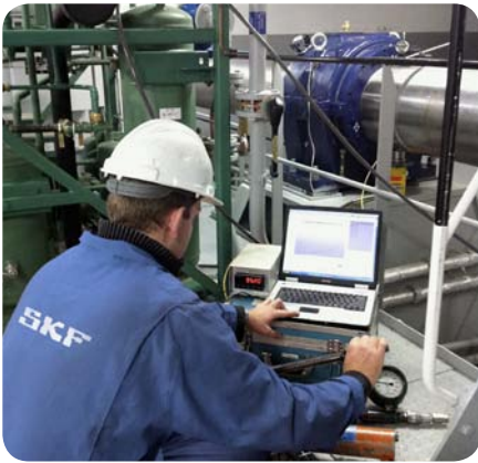
Shaft jack up test to check bearing loads and to validate theoretical calculated loads
